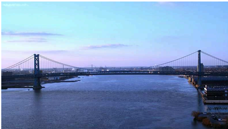
Fig. 1.3. Ben Franklin Bridge.
