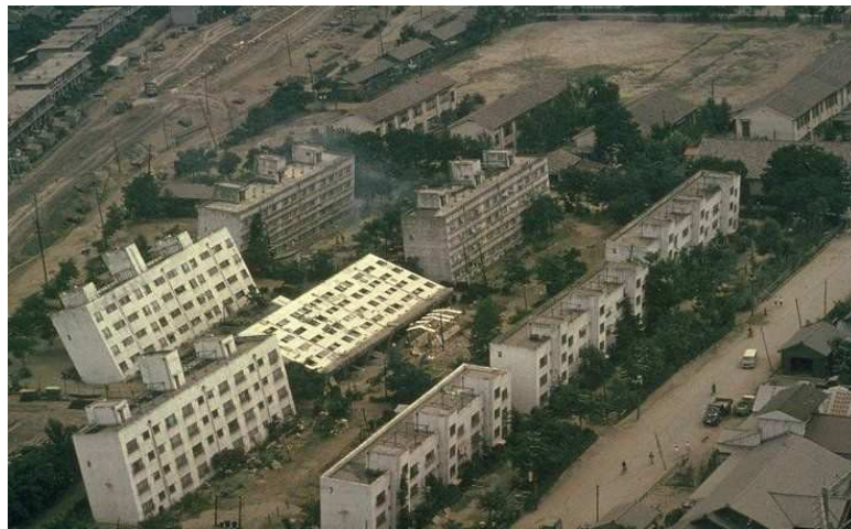
Fig 2.10: Liquefaction damage on building produced by the Niigata earthquake of June 16, 1964 (M= 7.5) ( http://www.usgs.gov/ ).
