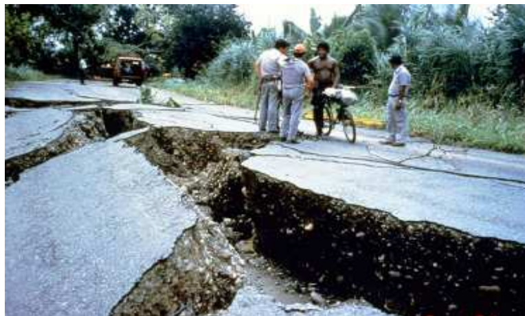
Fig 2.9: Lateral spreading (due to sediment liquefaction) caused by the 22 April 1991 Costa Rica Earthquake ( http://www.usgs.gov/ ).
