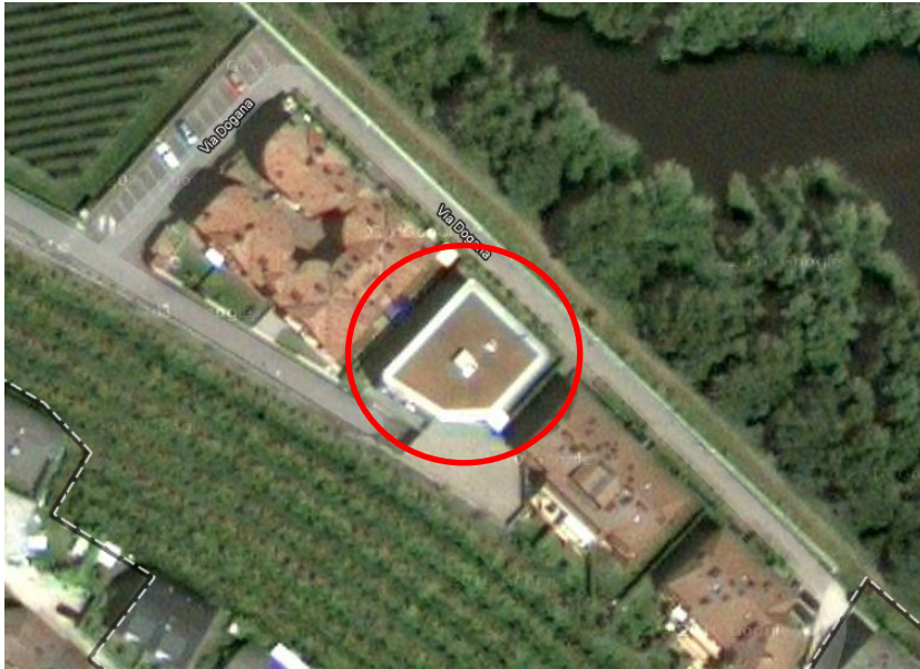
Fig. 3.5 top view of the building and its surrounding
