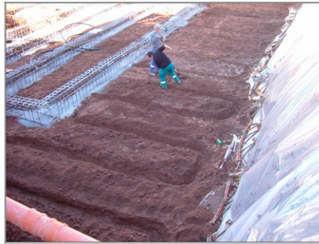
Fig. 3.17 Installation of geothermal probes
