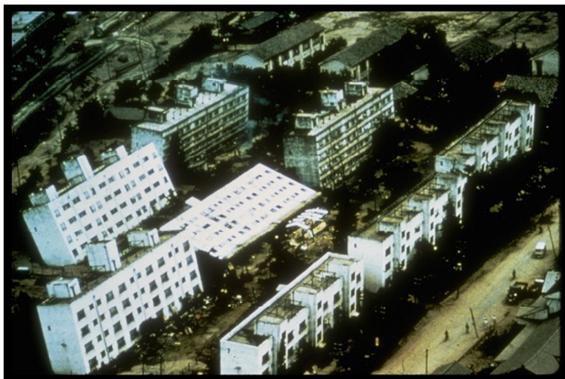
Figure 4. 10 Soil liquefaction and tilting during Niigata earthquake 1964 [ http://www.ce.washington.edu/~liquefaction/html/quakes/niigata/niigata.html ]
