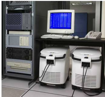
Fig. 1.9: Ballard's Airgen power systems. The rated power of each system is 1,2 kW and the system is already available on the consumer market.
