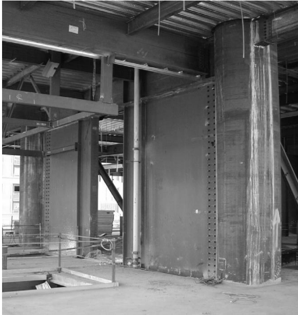
Figure 7.6 Steel Plate Shear Wall System
