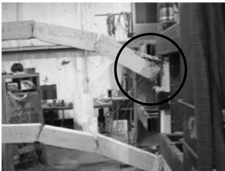
Figure 3.3 Tearing out of the stirrups is evident in the second level beam. [46]
