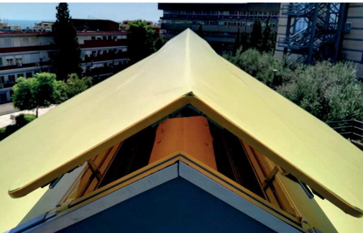
Figure 205 / Assembly of the ventilated roof ridge - On-site - University Campus, Catania (CT)
