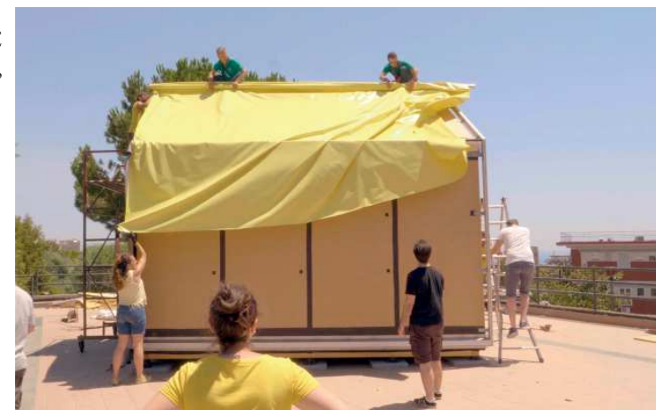
Figure 203 / Installation of the PVC textile - On-site - University Campus, Catania (CT)
