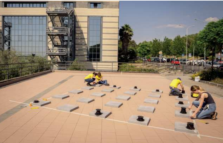
Figure 184/ Base footprint tracing and positioning of concrete blocks - On-site - University Campus, Catania (CT)
