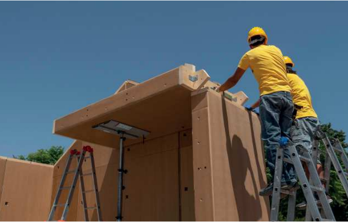
Figure 194/ Assembly of roof panels PACO 120 h250 cm by wooden joints and galvanized steel angular - On-site - University Campus, Catania (CT)
