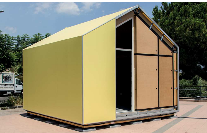
Figure 206 / Installation of window frame - On-site - University Campus, Catania (CT)
