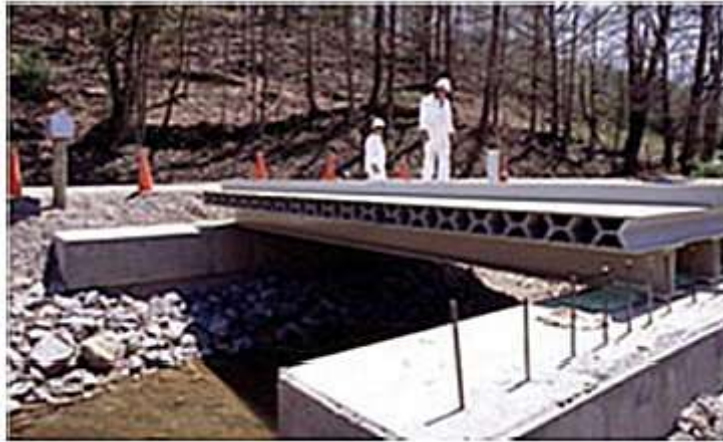
Fig. 1.63 Laurel Lick Bridge, 1997 West Virginia
