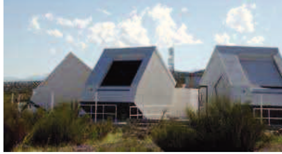
Figure 3.8: Photo of the three HEAT buildings in tilted mode.
