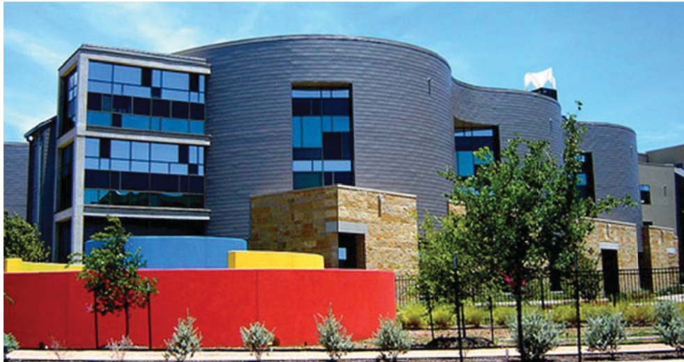
Figura 6.1.1 – Dell Children's Hospital.
