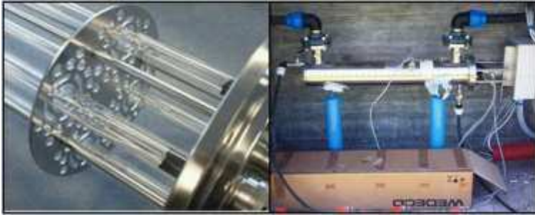
Figure 11: UV system, mod. WEDECO AG, LBX 10 used in ARU2 treatment system
