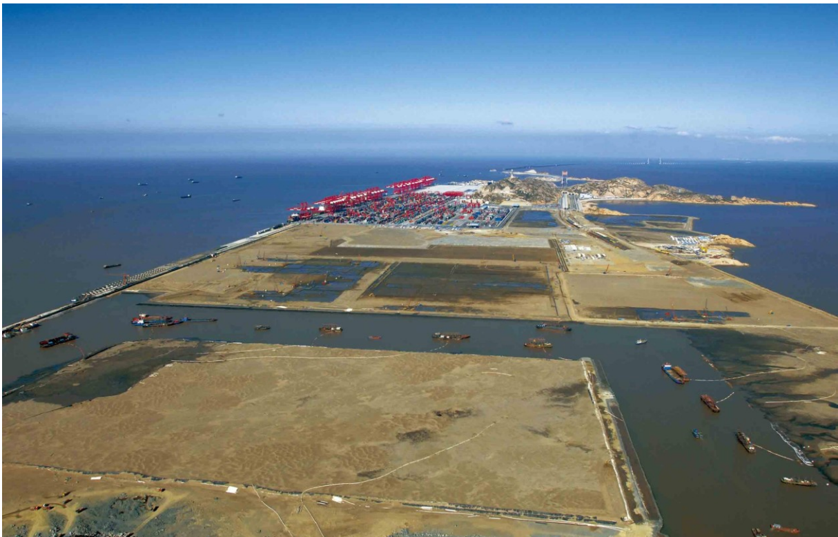
Figura 58 - Shanghai, Yangshan Deepwater
