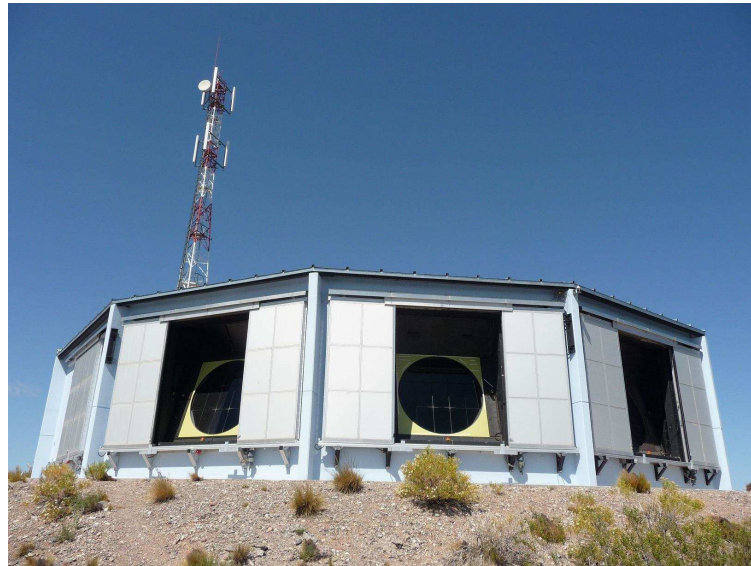
FIGURE 7.1: FD building at Los Leones; behind the building is a communication tower.
