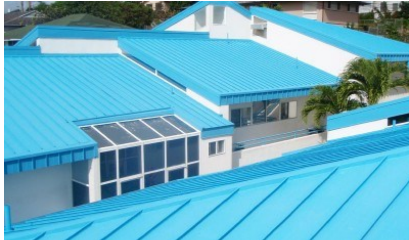
FIGURE 2.1: View of cool roofs in Honolulu, Hawaii [Internet]
