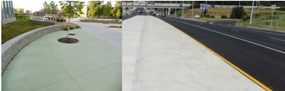
FIGURE 3.6: Cool pavements (on the left) and cool asphalt (on the right) [Internet]
