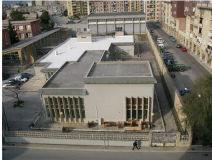
FIGURE 3.16: Cool roof application in a school building in Trapani [26]
