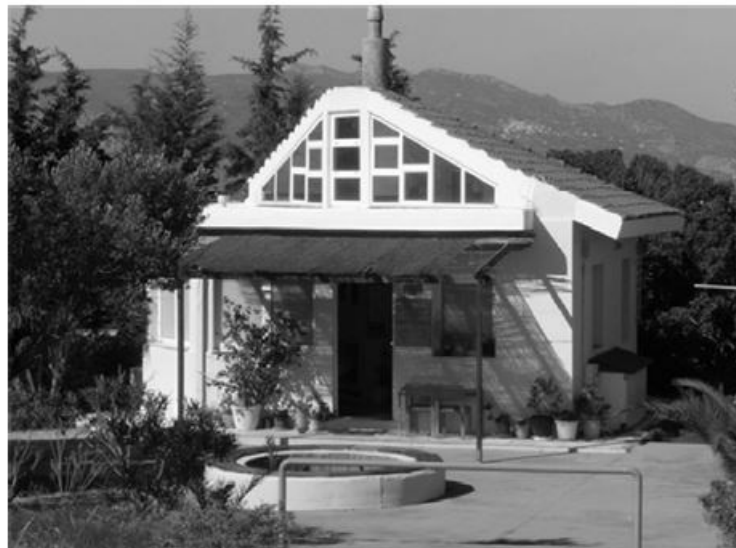
FIGURE 3.12: The house investigated for the Iraklion case study [24]
